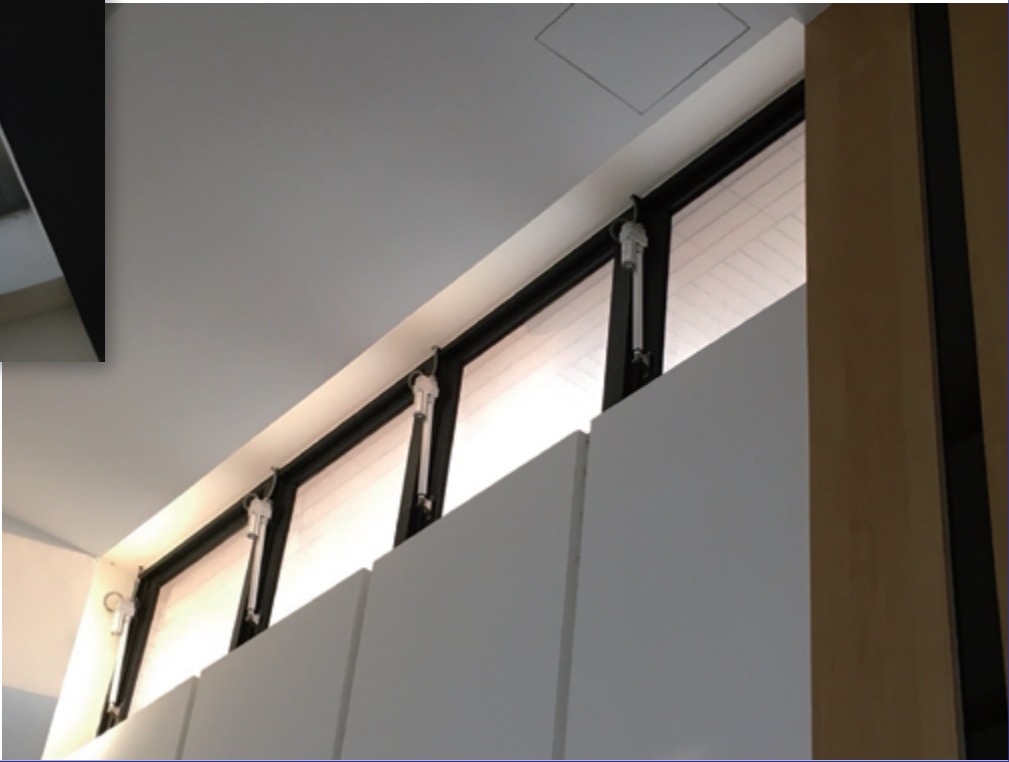
KST-E01 for skylight windows. For both inducing natural light and fresh air.
