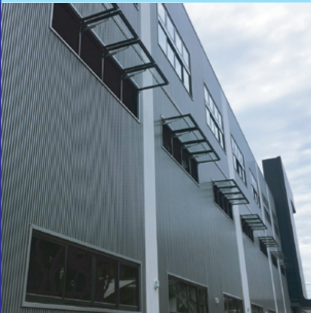
@Factory. For smoke ventilation, daily natural ventilation and parallel control a row of windows.
