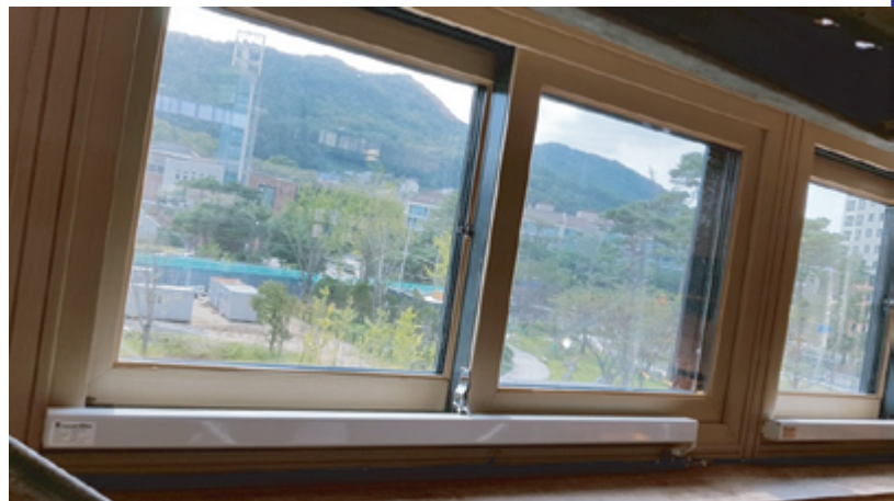
@ Gym of elementary school. High windows for natural ventilation. With parallel operation with remote controller.
