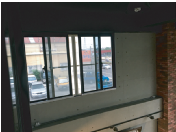
@ Workshop. Opening high sliding windows for natural ventilation by remote controller.
