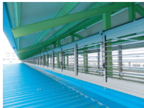
@Factory. For opening a row of electric jalousie windows with remote control.
